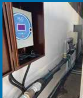
Electronic water conditioner at Cooling Tower 1
