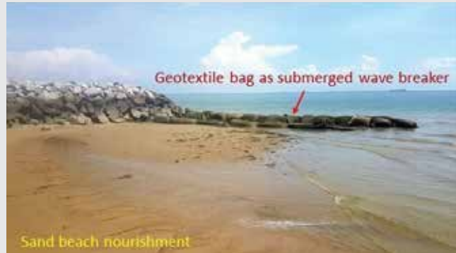
The submerged breakwater will control and reduce beach erosion by sand nourishment which increases the beach area and coastline gradually (July 2020).
