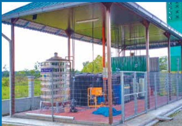
Fabrication of water nanofiltration system at Masjid Desa Aman, Kedah.
